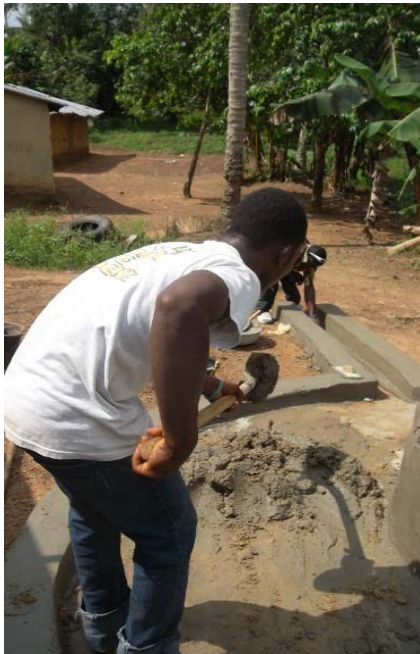
Project in process.
